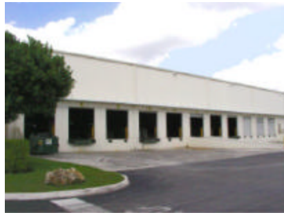
Bays of the warehouse
